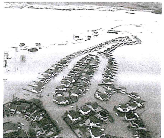
New Year's flood in downtown Reno. Downtown Reno and the Hidden Valley are inundated during the New Year's flood of 1997. Planning and zoning board restrict permanent construction in flood-prone areas. Photo by Martin Fowler, Reno Gazette Journal
